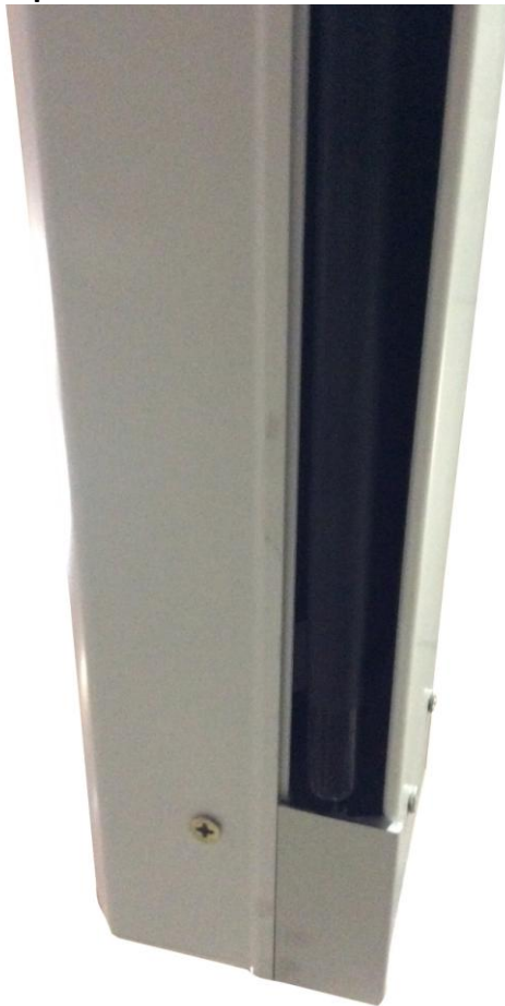
Close up of bottom
